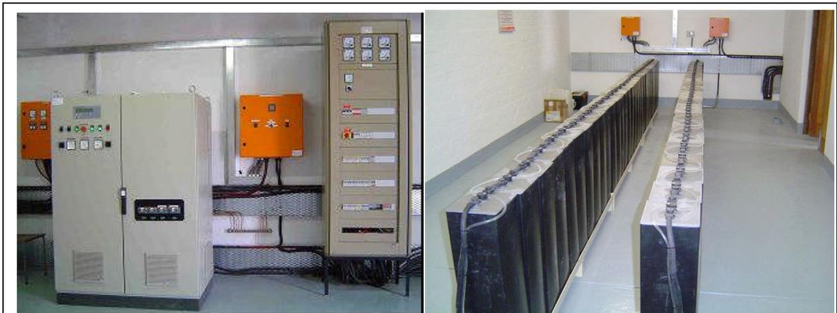
**Figure 3: The Gobabeb hybrid electricity system's operation room, and 200 kWh battery bank**
